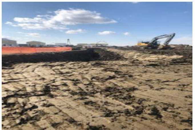
Bell hole being backfilled at tie in – km 179+650 – Oct 5, 2018
