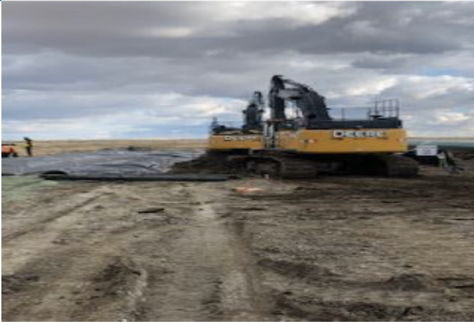
Excavator digging out tie in plug – SF 92 – Oct 3, 2018
