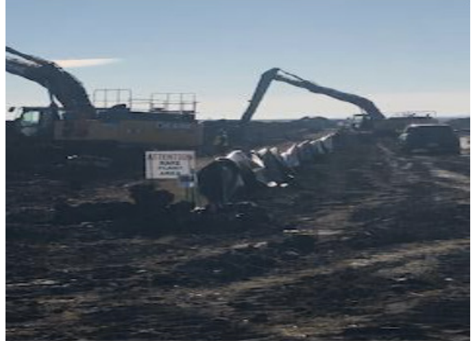
Rare plant area being backfilled – km 153+200 – Oct 6, 2018
