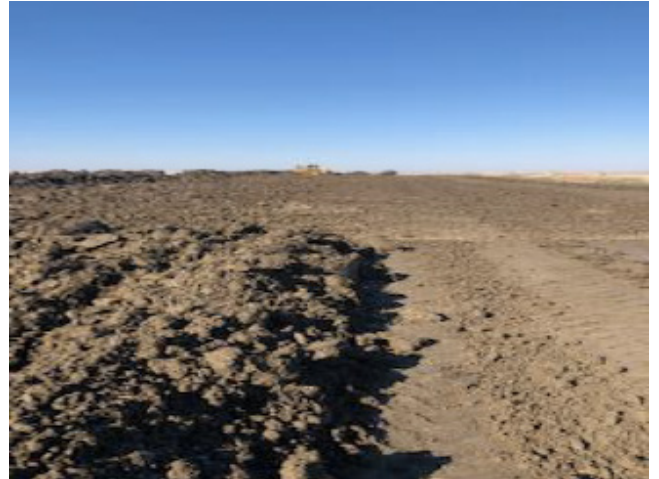
Topsoil being stripped – km 251+700 – Oct 6, 2018
