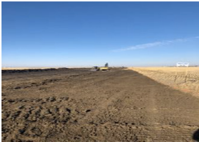
ROW being stripped - km 263+500 – Oct 6, 2018
