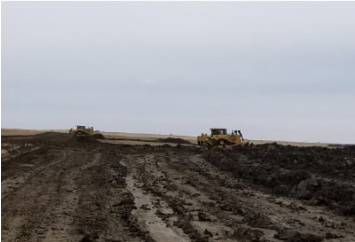
Spill pile from mainline ditcher - km 154+500 – Oct 4, 2018
