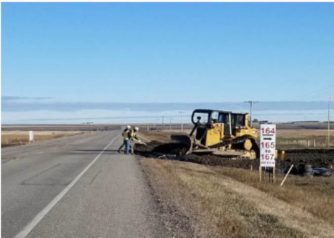
Building ramp – km 259+141 – Sept 30, 2018
