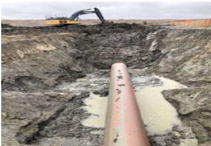
Shade and backfill – Oct 1, 2018
