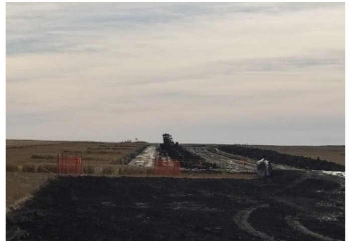
Grader moving dirt– km 247+355 – Sept 30, 2018
