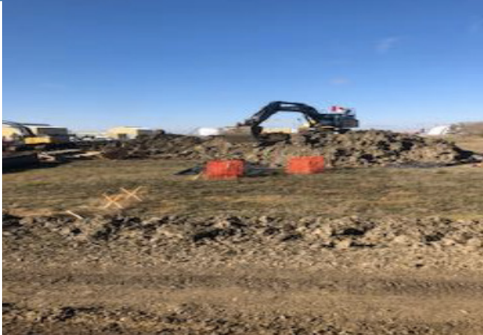
Backfill at tie in - km 179+836 – Oct 5, 2018
