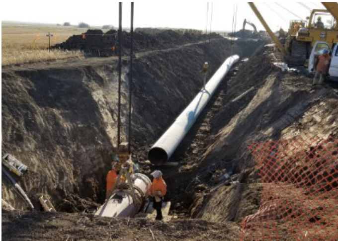
Prepping tie in - km 149+940 – Oct 6, 2018
