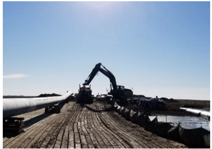
Offloading pipe weights – km 153+100 – Oct 6, 2018
