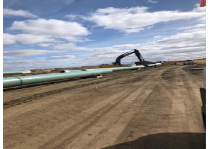
Excavator transitioning welds – km 182+900 –Sept 30, 2018
