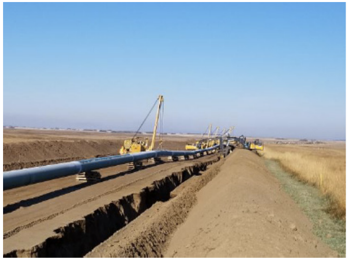
Lowering in – km 155+400 – Oct 5, 2018
