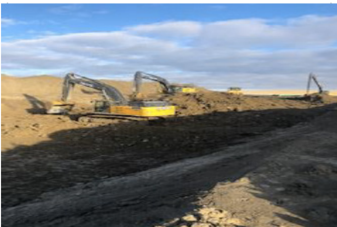
Digging bore bay – Km193+075 – Sept 30, 2018
