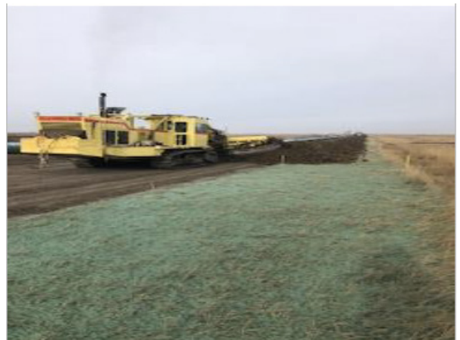
Digging ditch on mainline– km 154+900 – Oct 4, 2018
