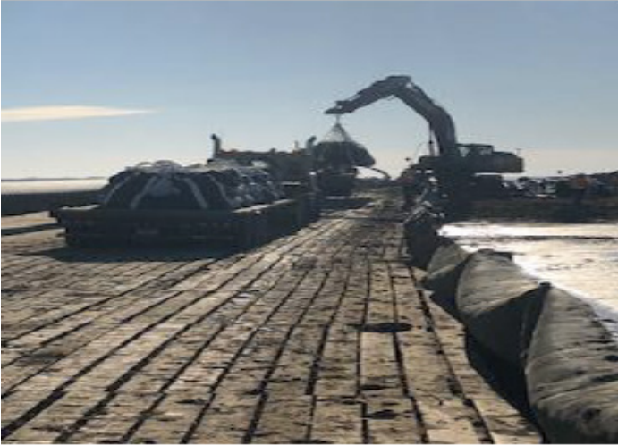
Excavator unloading swamp weights - km 153+100 – Oct 6, 2018
