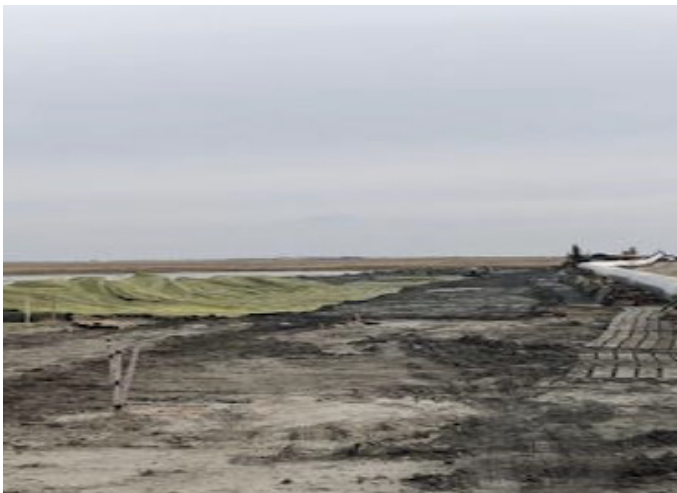
Crew laying geo tec at Heritage site – SF 92 – Oct 4, 2018
