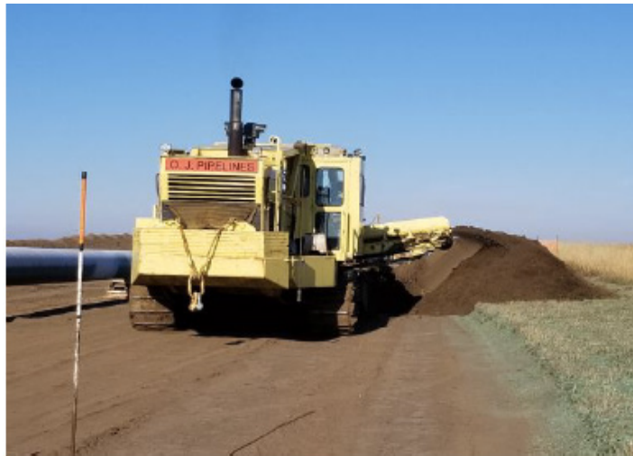
Ditching wheel - km 155+800 – Oct 5, 2018
