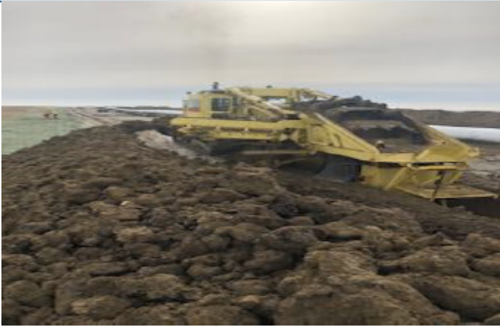
Spill pile from mainline ditcher - km 154+500 – Oct 4, 2018
