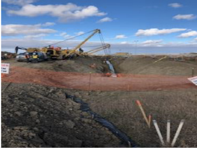
Tie in at bore – SF 91 – Sept 30, 2018
